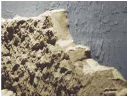
*Material buildup on interior wall of cement silo restricts material flow, reduces storage capacity, and impacts finished product quality.*
